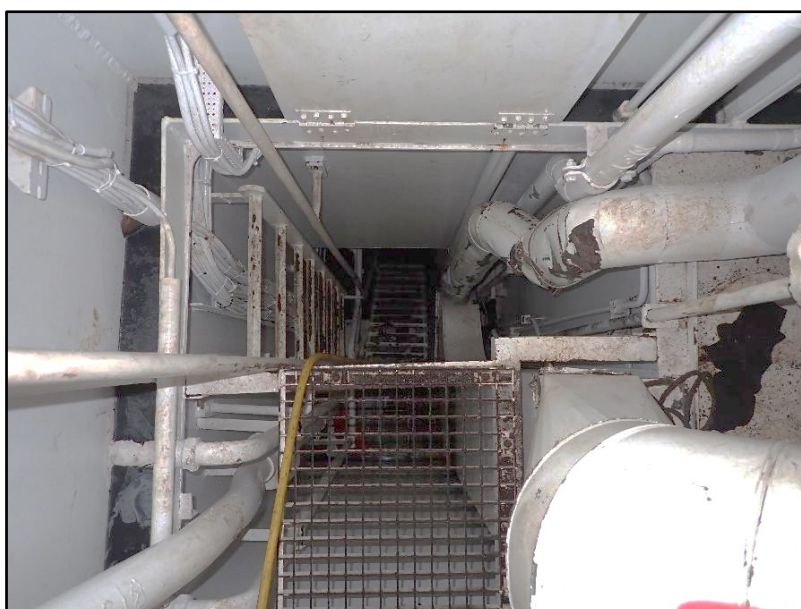
Figure 5: Access to bow thruster room, viewed from top of ladder looking down
