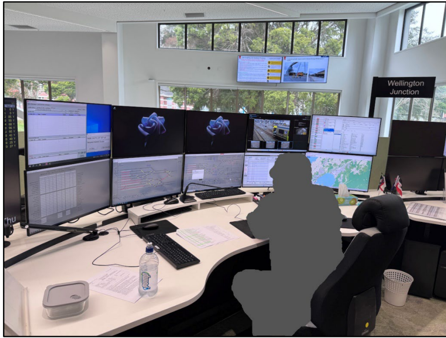
Figure 3: Wellington Junction train control desk
