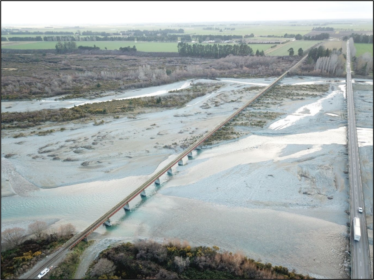
Figure 1: Bridge 57 Main South Line (July 2020) (Credit: KiwiRail)
