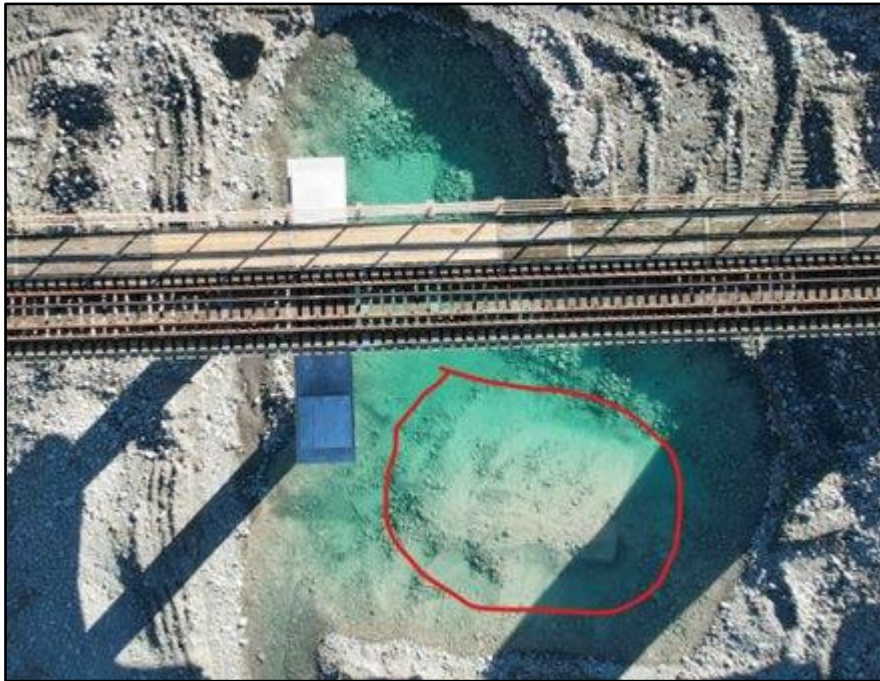
Figure 15: Final location of Pier 8
