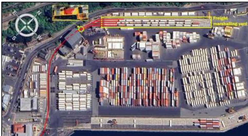
Figure 3: Port Otago rail storage facility
