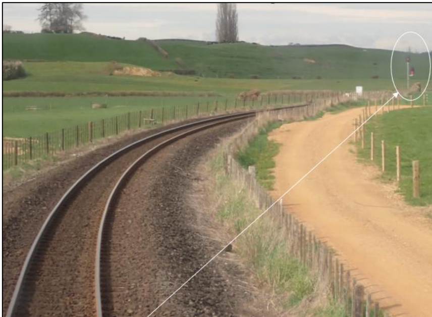
Figure 22: Signal sighting of intermediate signal on the right-hand bend
