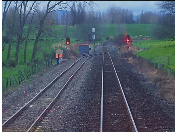
Figure 9: Crossing loop signal (signal 4LB) on the left and exit signal (signal 4LA) on the right
