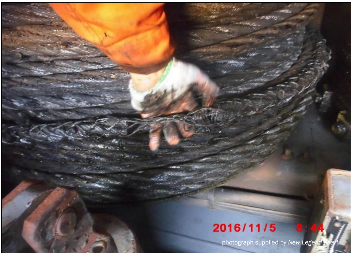
Figure 3 Cable sock joining the old wire and the replacement wire
