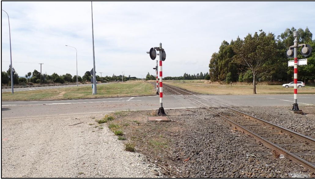
Figure 6: Protection devices in place at the crossing
