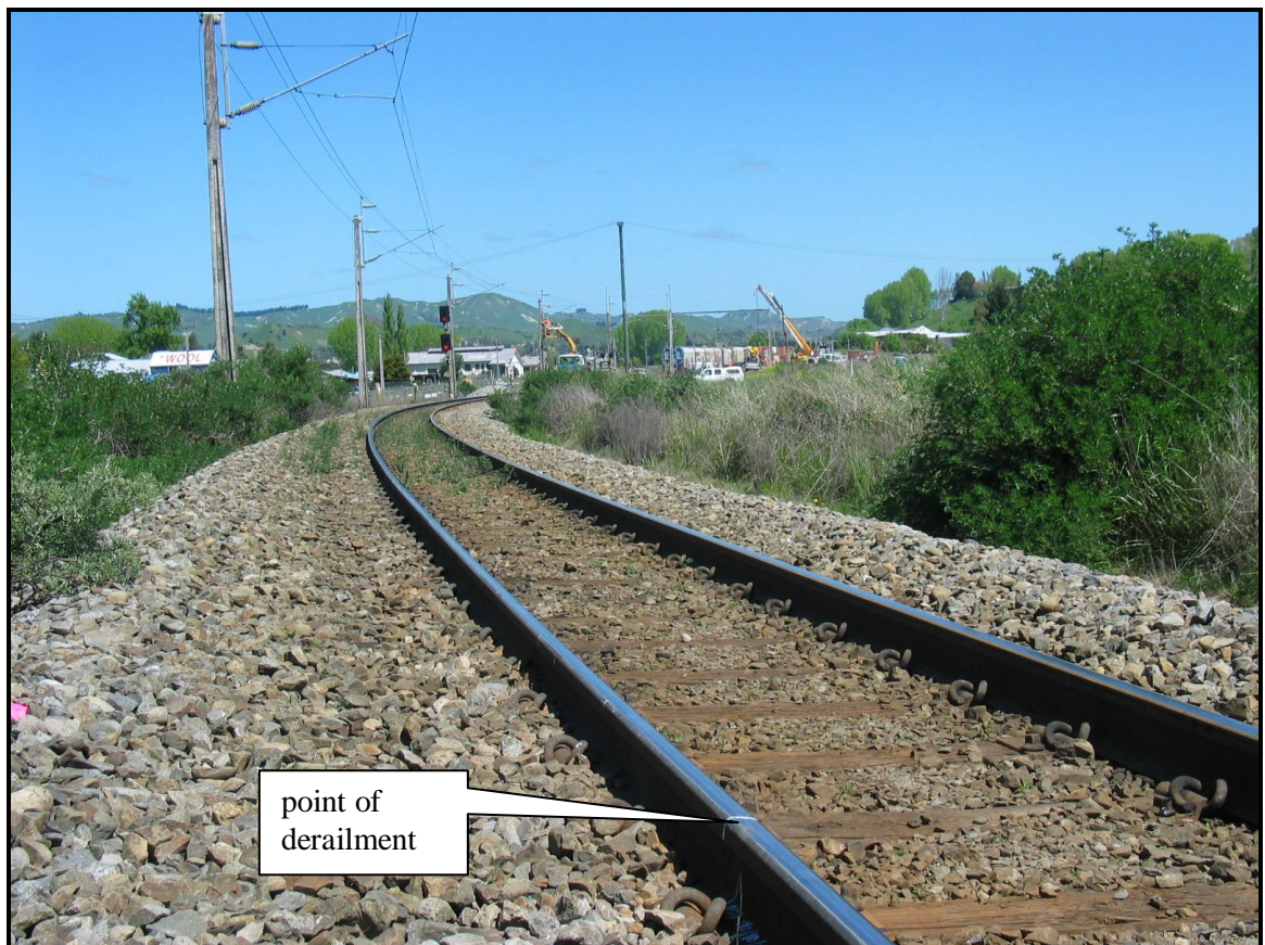
Figure 1 Track formation at the point of derailment
