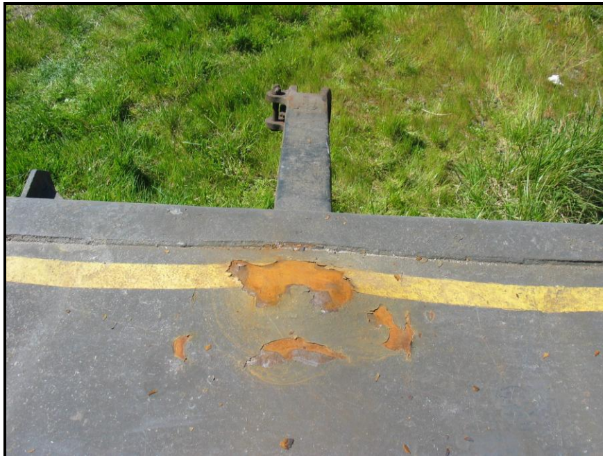
Figure 7 Deck at the trailing end of wagon PKH34
