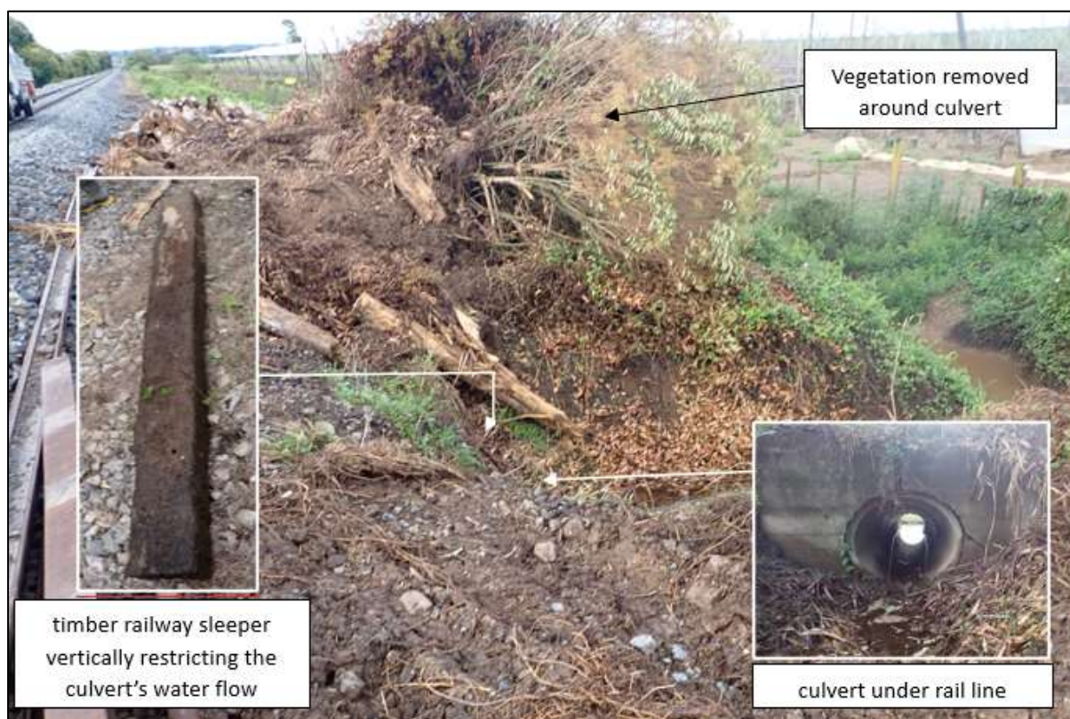
Figure 23: Western entrance of culvert
