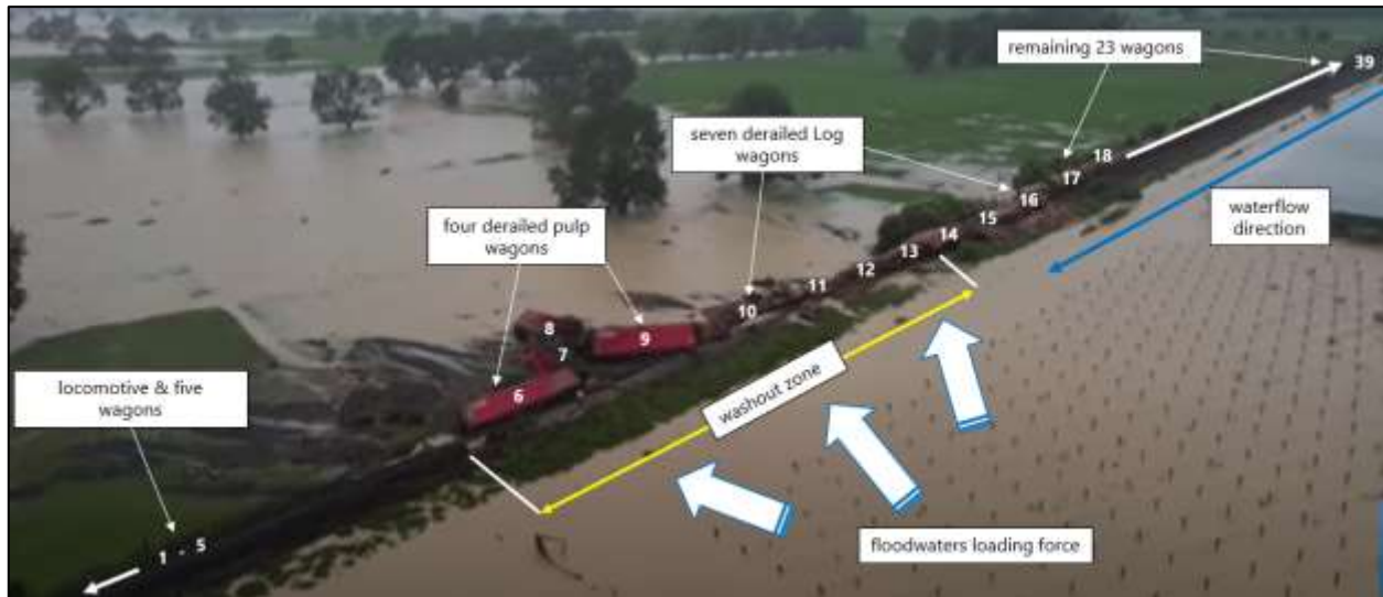
Figure 10: Derailment site from west side (drone footage taken at 0800 on 29 January 2023)
