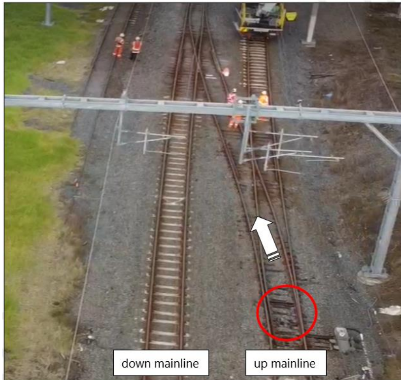
Figure 14: Crossover points set to bring the locomotive from the up mainline onto the down mainline.
