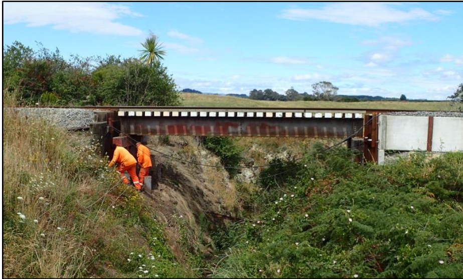
Figure 6 Location of bridge work group members when the train crossed Bridge 107
