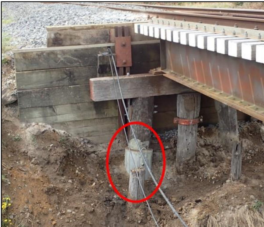
Figure 2 The repaired section of bridge support
