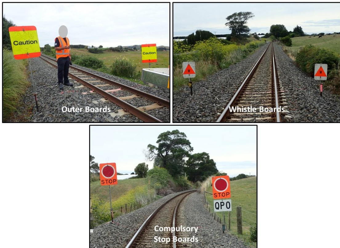
Figure 4 The warning boards and compulsory stop boards for the worksite
