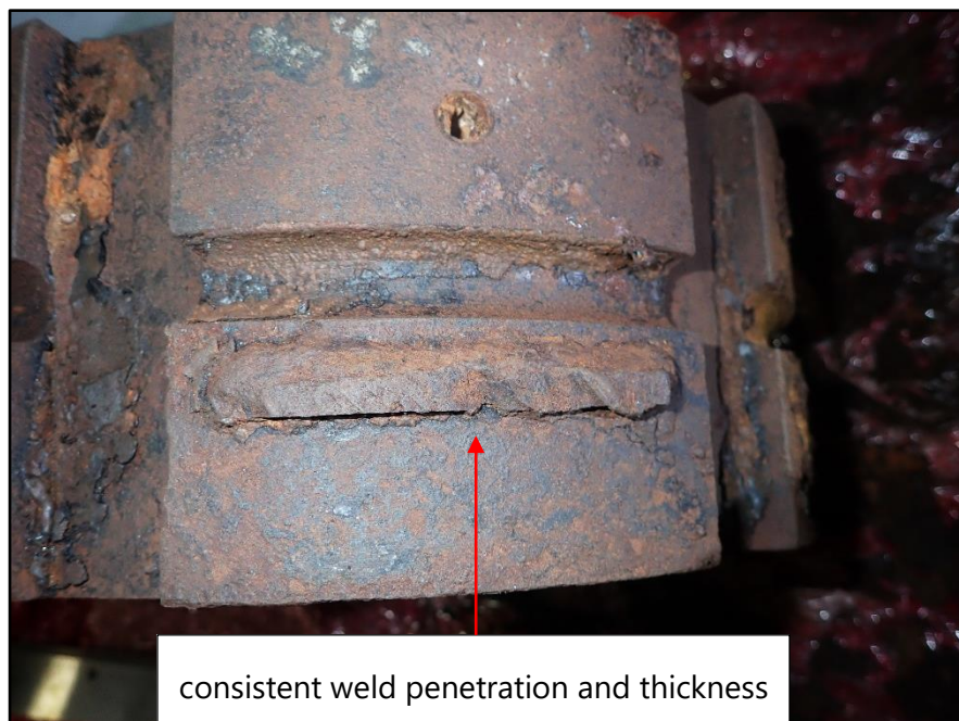
Figure 20: Original 2003 weld connecting pintle stopper to side of nut
