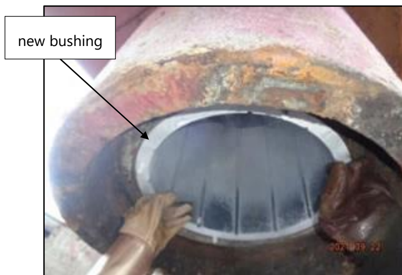
Figure 9: Pintle removed, new bushing installed (viewed from below the gudgeon) 2021 (Credit: Shanhaiguan Shipbuilding Industry Co Ltd)
