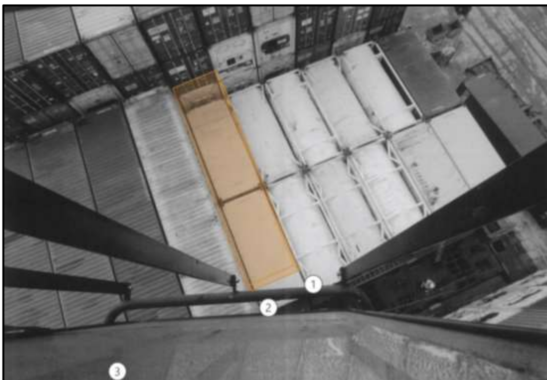
Figure 12: View looking down from outside the number three crane cab window
