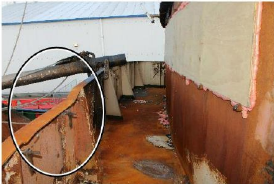
Photo 6: The circle indicates the warping of the gunnel in front of the bridge windows. Note: this is all on the port side of the bridge.
