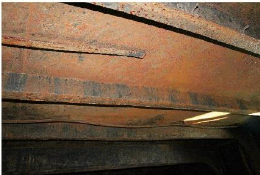
Photo 14: Shows the burn pattern on the ceiling in a line between the porthole and the rubbish bin.
