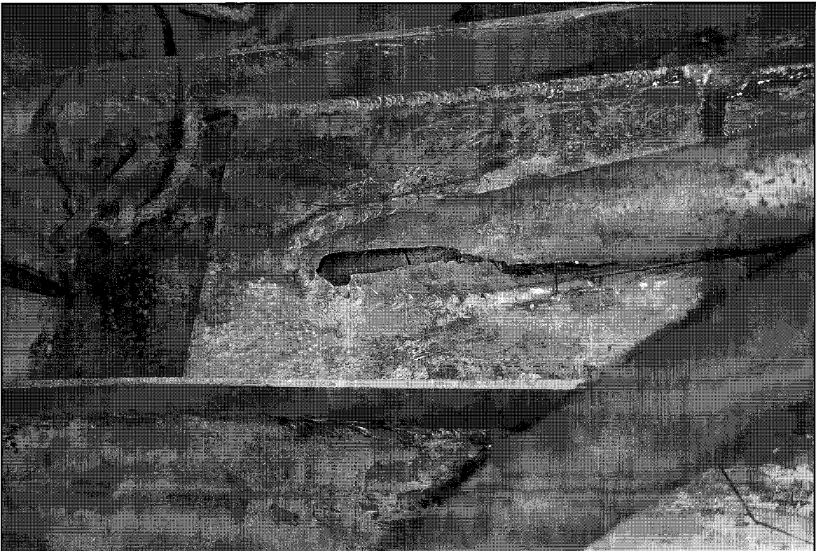
Hull penetration from the outboard side
