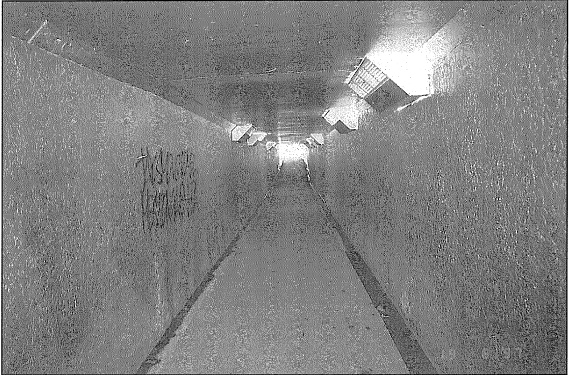
Figure 4 Pedestrian subway looking east to Glen Innes shopping centre exit
