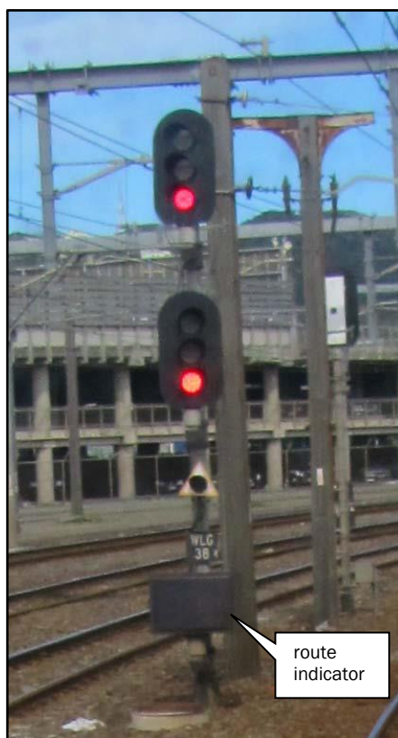
Figure 1 A route indicator
