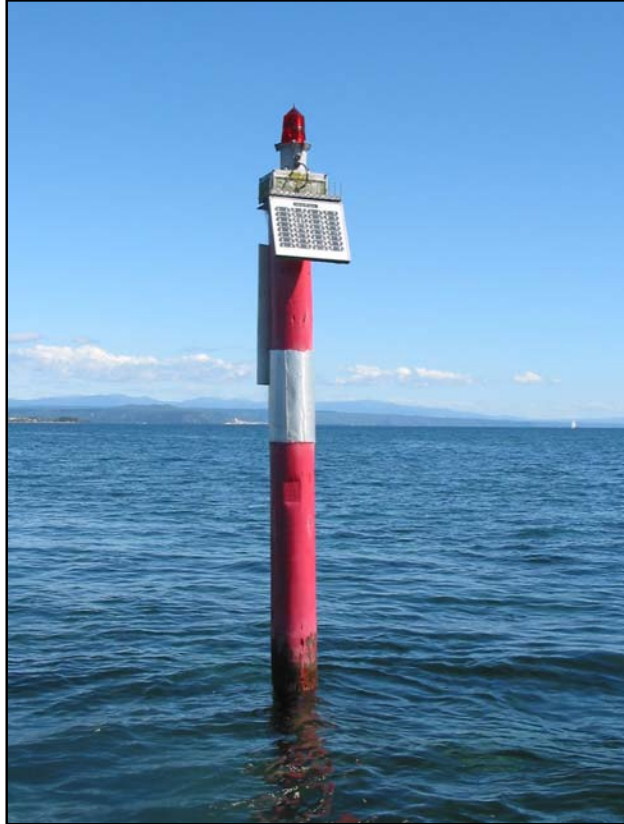
Figure 5 Port-hand entrance channel beacon
