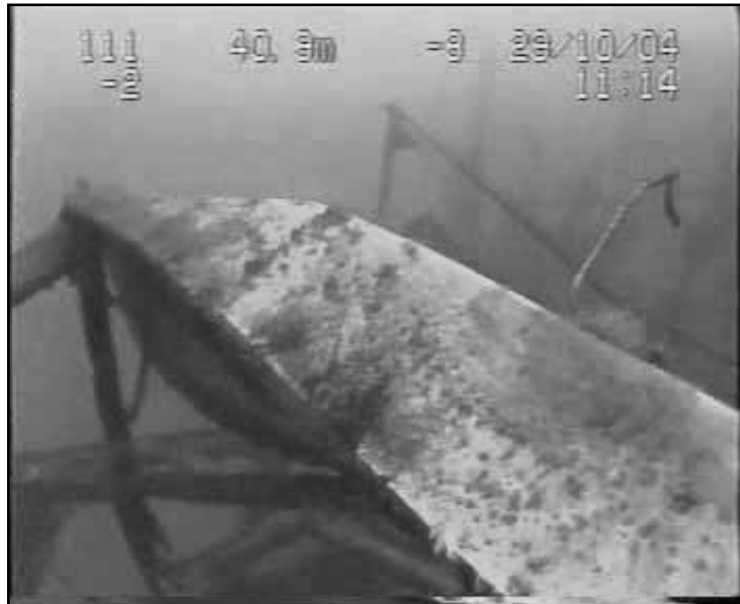
Figure 15 Damaged awning structure
