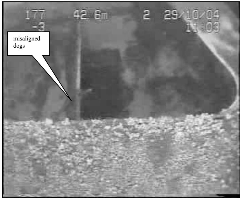
Figure 8 Port watertight door
