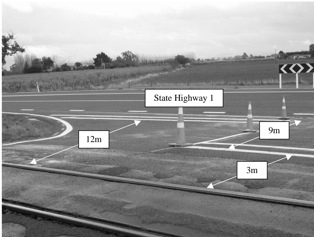
Figure 4 The State Highway 1 side of the level crossing showing the limit lines for traffic approaching the intersection and approaching the level crossing
