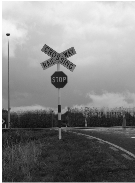
Figure 3 The Compulsory Stop sign on the Vickerman Street side of the level crossing
