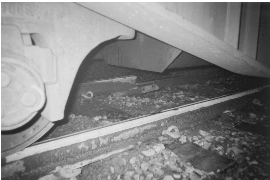
Figure 2 Two views of the closure rail east joint as found following the derailment (Train 842 still in position)
