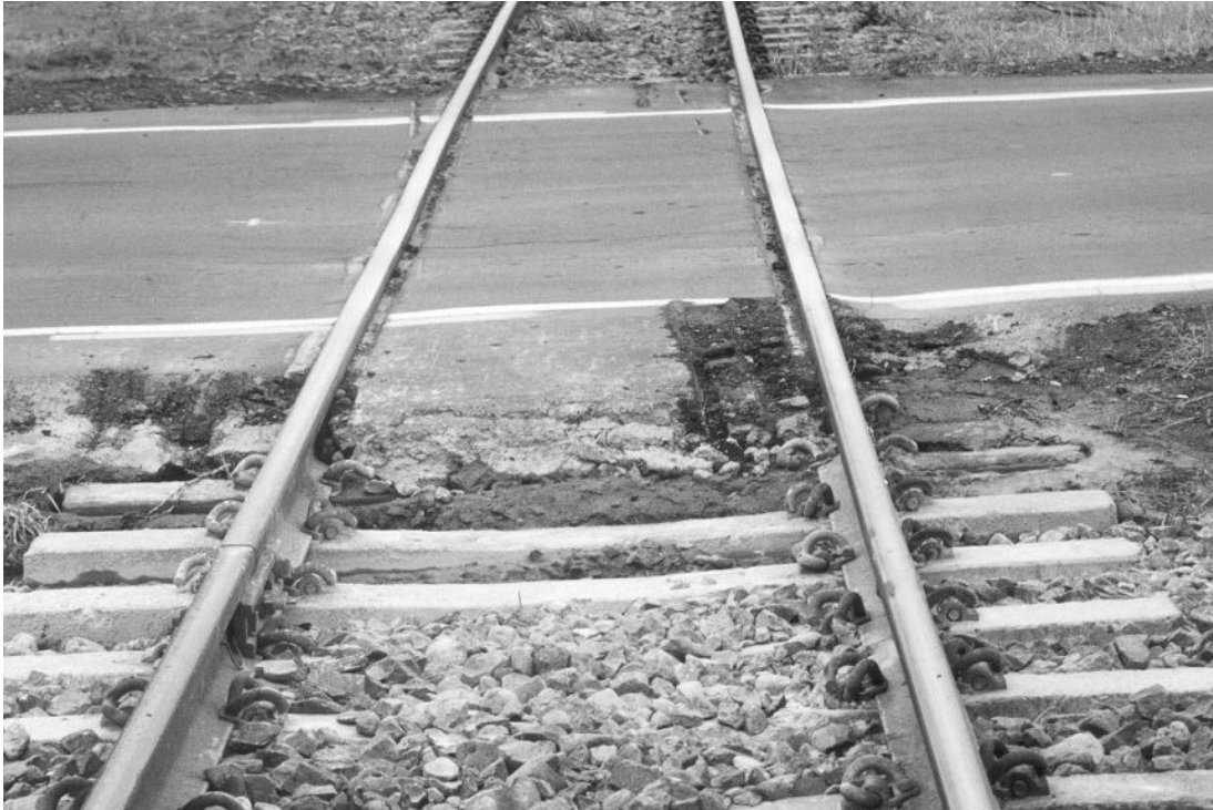
Figure 3 The northern edge of Otaihanga Road level crossing
