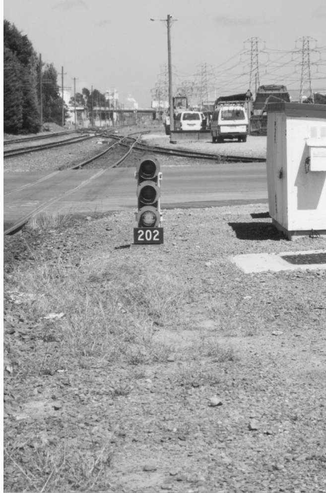
Figure 3 Signal 202 with Points 206 and 207 and Curletts Road overbridge in the background
