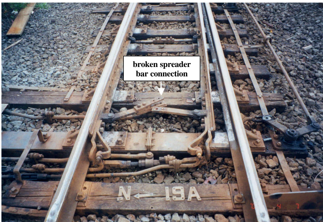
Figure 1 Looking north at the up main to loop points following the derailment
